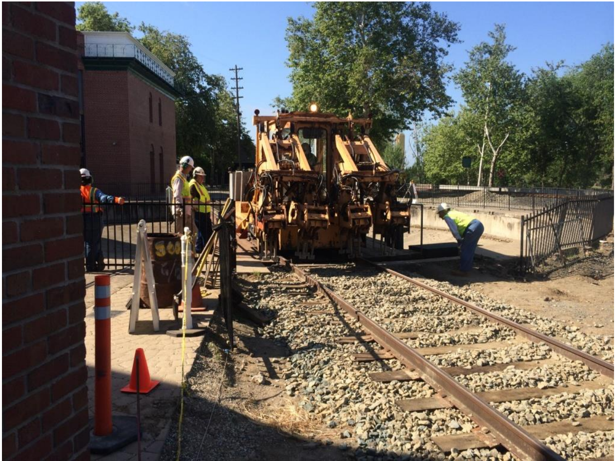
Now it's the tamper's turn to shake things up
